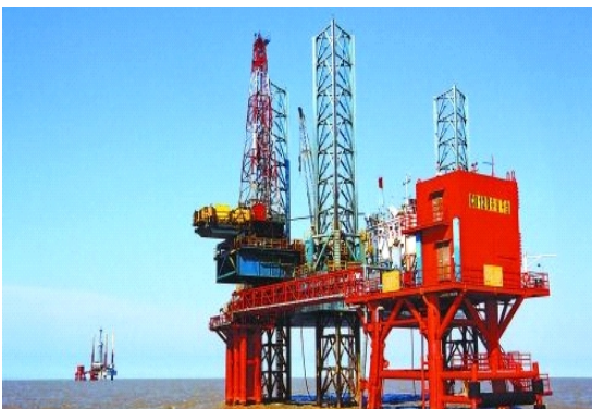
Oil field communication system
